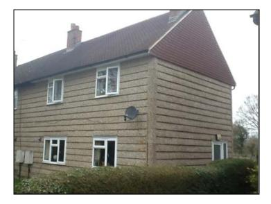
Airey's were a fast-build system to help ease the housing shortage, following WW2. Due to problems with the concrete supporting frame, they were structurally repaired, on a nation-wide scale, in the late 1980's or early 1990's. The external walls were provided with some insulation, in the form of insulated plasterboard, on the inside. Even though improved however, the thermal performance is still inferior, when compared to traditional external wall construction.
